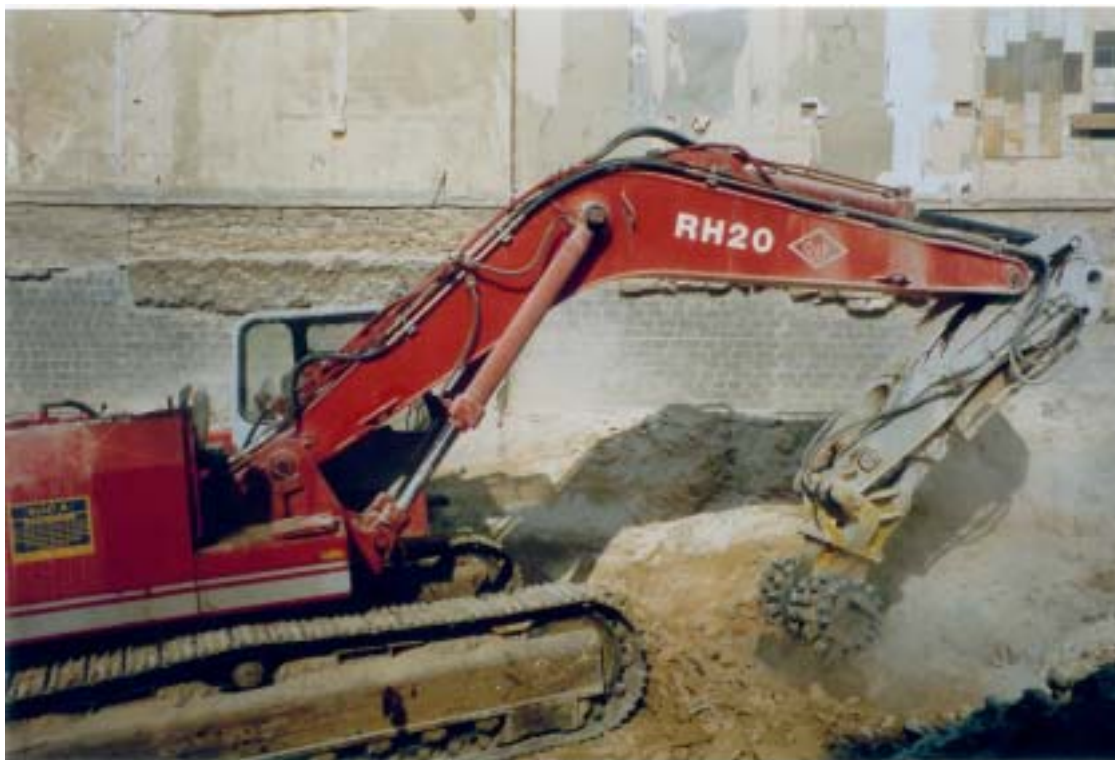
ETH 50 mounted to an O&K RH 20 excavator
